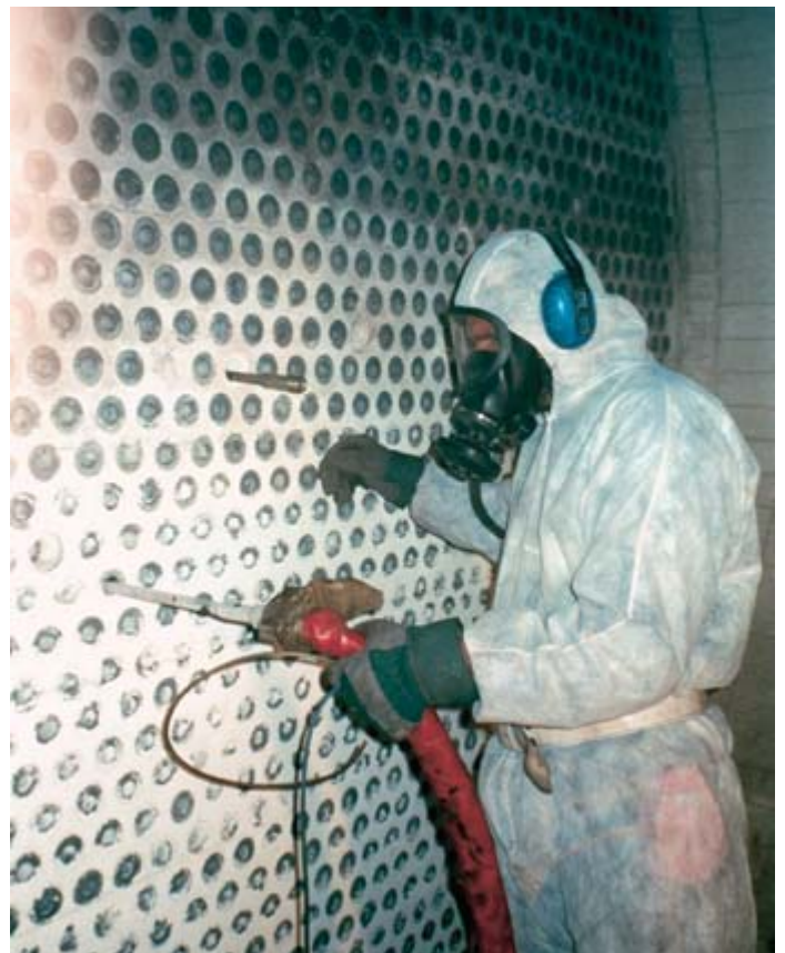
In some cases, gas masks are highly recommended – e.g. when cleaning heat exchangers and harmful materials are blasted loose.
